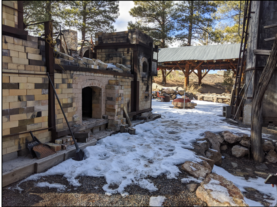
Figure 1-5: Front View of the Kiln Looking North
